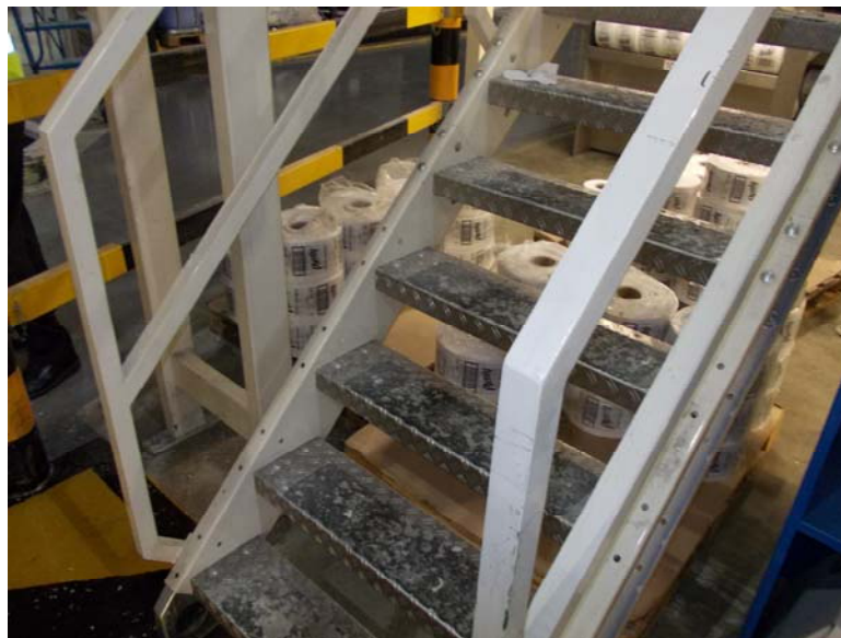
Nearby flight, no nosing highlight, small goings, worn grip pads
