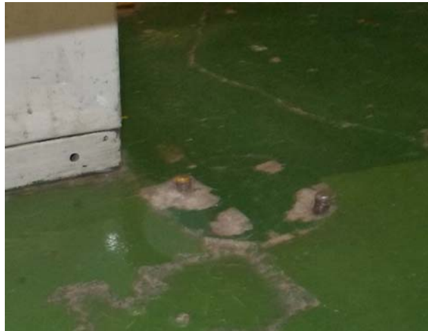
Bolts left in walkway after barrier has been moved
