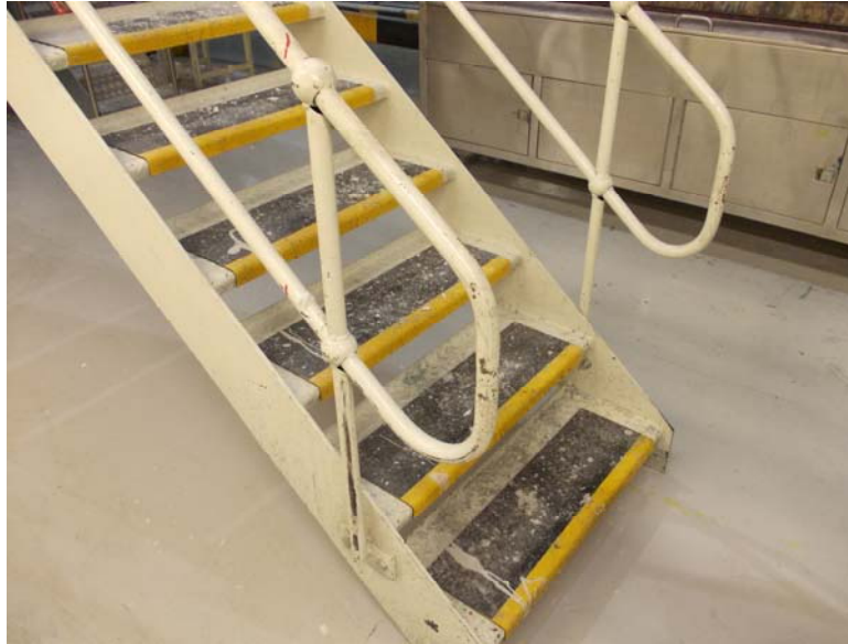
An example of good practice, anti slip treads with a clearly marked nosing
