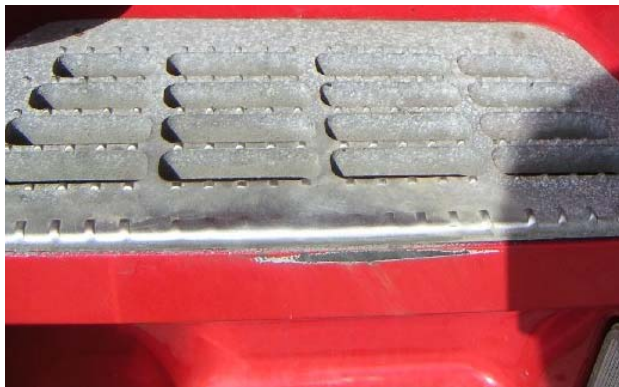
Severely worn step tread offering little slip resistance
