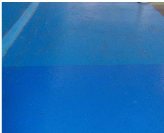
Example of inconsistency in floor finish, part way along a walkway
