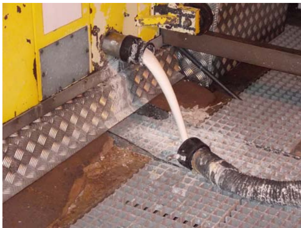
Composite drain covers need to be installed with the rough surface upwards
