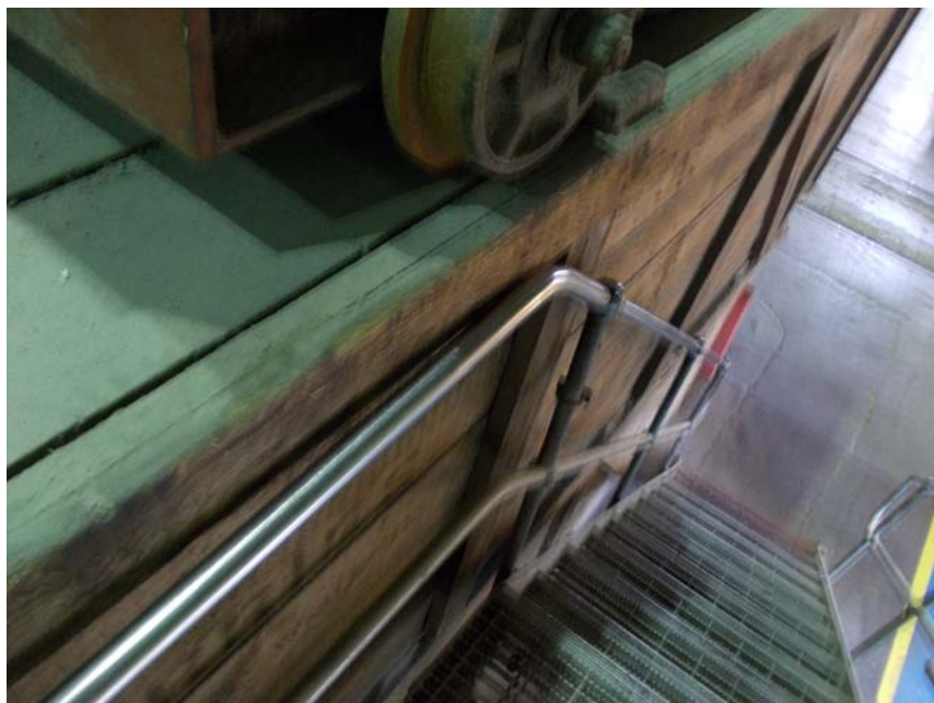
Handrail compromised by storage of crates
