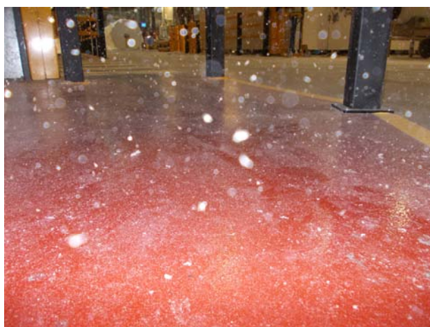
Example of dust contamination
