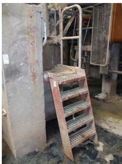
Steep plant access steps where space would allow larger going
